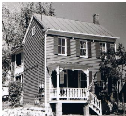
Ca. 1985 After restoration following Revolving Fund purchase
